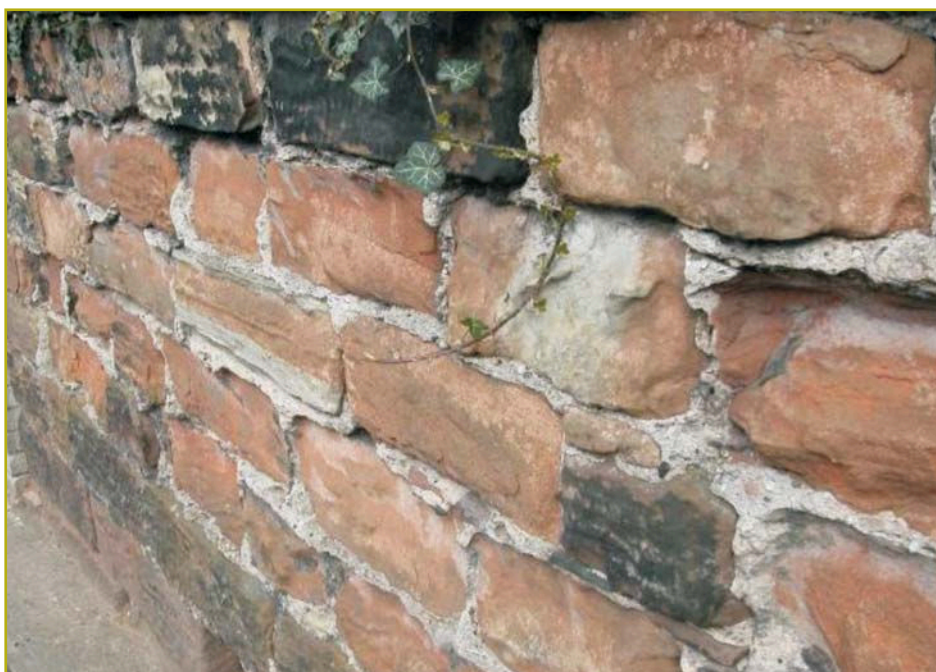
Figure 34: Examples of hard cement mortar damaging stonework: (above) Hard cementitious mortar joints damaging a stone boundary wall and (right) Damaging and unattractive cementitious render repairs
