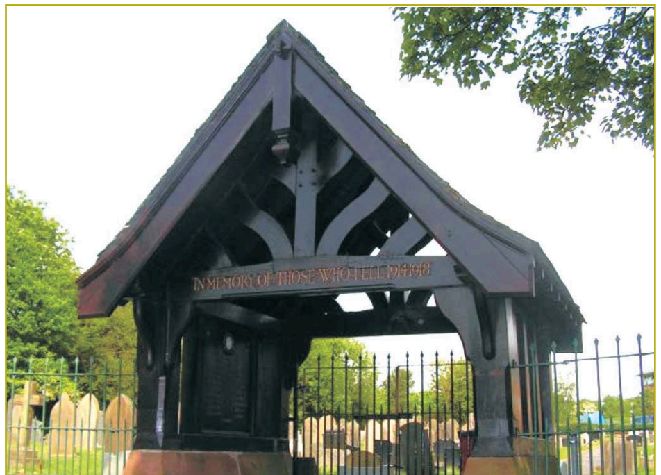
Figure 18a: Lych Gate marking the entrance to Halton Cemetery from Holt Lane
