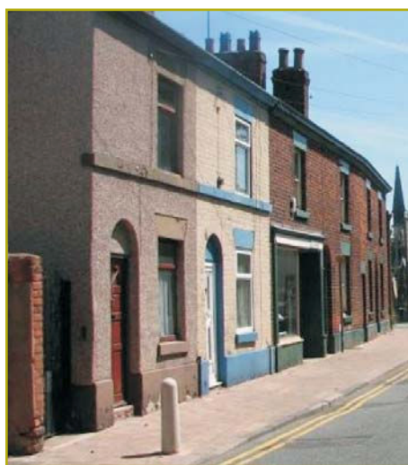
Figure 36: The effects of stone cladding and pebbledashing on individual housing and the overall street scene
