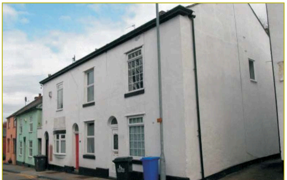
Figure 25: Examples of architectural styles present within Halton Village: (clockwise from top Elizabethan; Georgian; Victorian terraces and a Victorian house.
