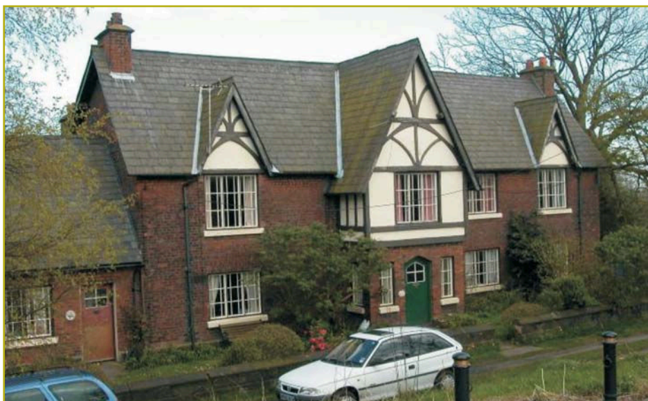
Figure 21b: Hill House, Castle Road
